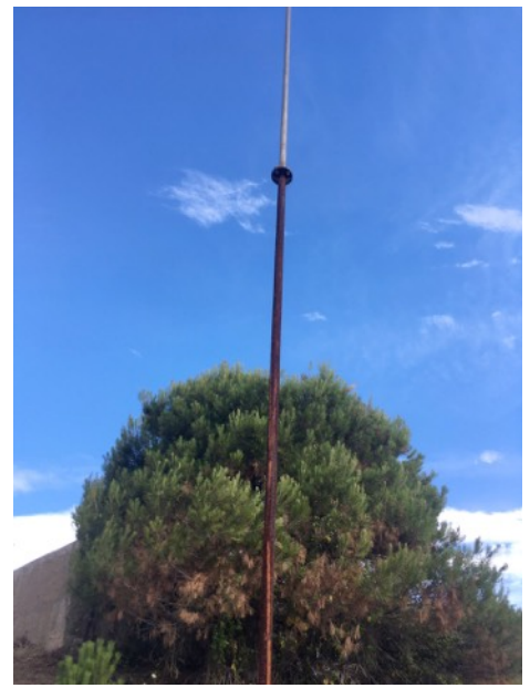
Pipes being extracted from well.
